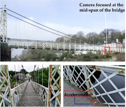
Fig. 1. Daly's bridge: general view (from west and looking across north) and position of a wireless accelerometer for the trials
