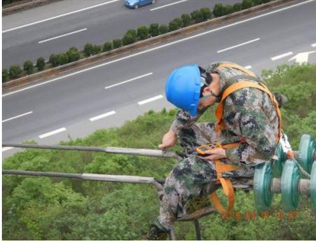
**Fig. 3.** Ultrasonic inspection of the thickness of the aluminum layer on the crimping surface
