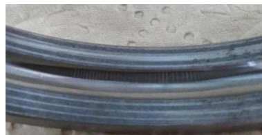
b) Axis current outer ring failure
