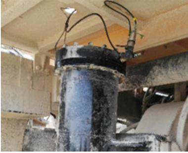
**Fig. 5.** Installation location of the acceleration sensor
