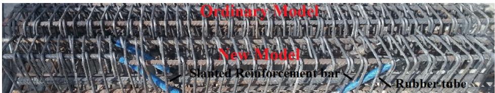
Fig. 4. Reinforcements in the ordinary and new models (proposed models)
