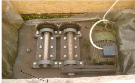
Fig. 6. Centrifugal direct-action vibrator in container storage: 1 – location of accelerometer
