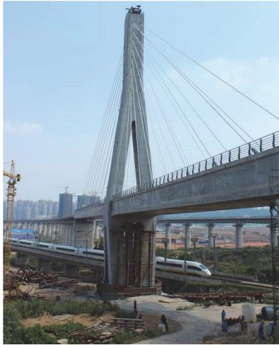
Fig. 1. Built single tower cable-stayed bridge
