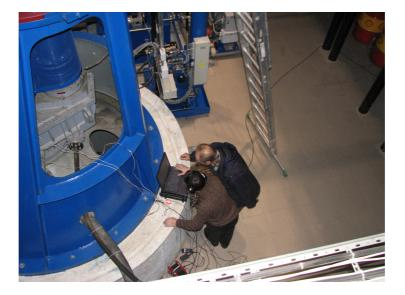
Fig. 1. Measurement of vibrations of the machinery at Balskai hydroelectric power station
