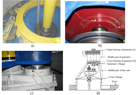
**Fig. 2.** Mounting points of transducers while measuring the vibrations of hydromachinery bearings: a) vibrations of turbine bearing in the radial direction (1) and vibrations of turbine cover in the vertical (2) direction; b) vibrations of generator bearing in the X direction; c) reducer vibrations in the radial (1) direction; d) measurement points of vibrations along the hydromachine
